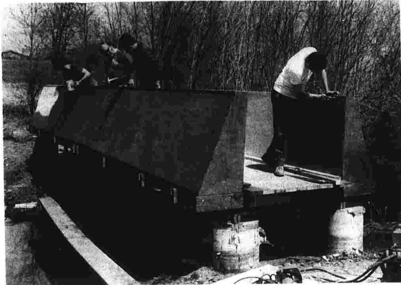
Jaycee Bridge Builders at Work
